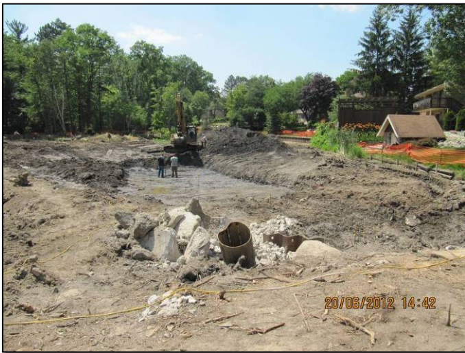
June 20, 2012: Excavation of proposed channel
