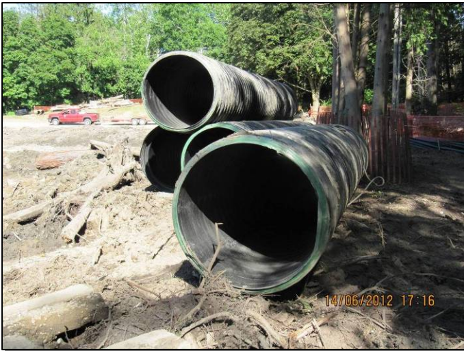
June 14, 2012: Pipe onsite for bypass flume
