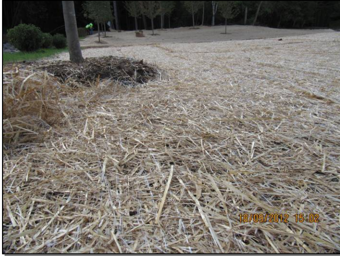
September 18, 2012: Erosion Control Blanket
