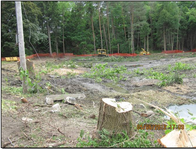
June 5, 2012: Looking south across pond; cleared and dredged area
