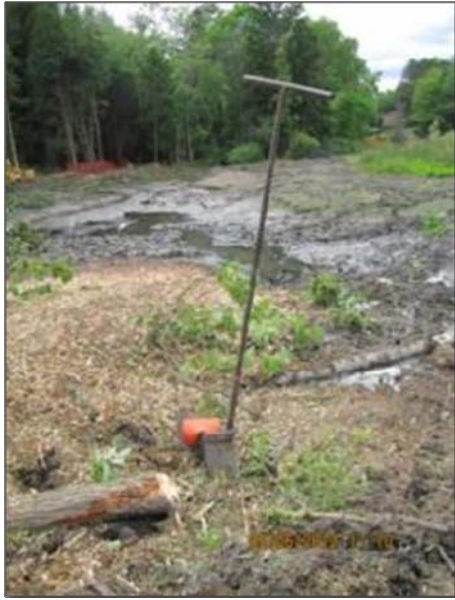
Existing bypass valve opened
