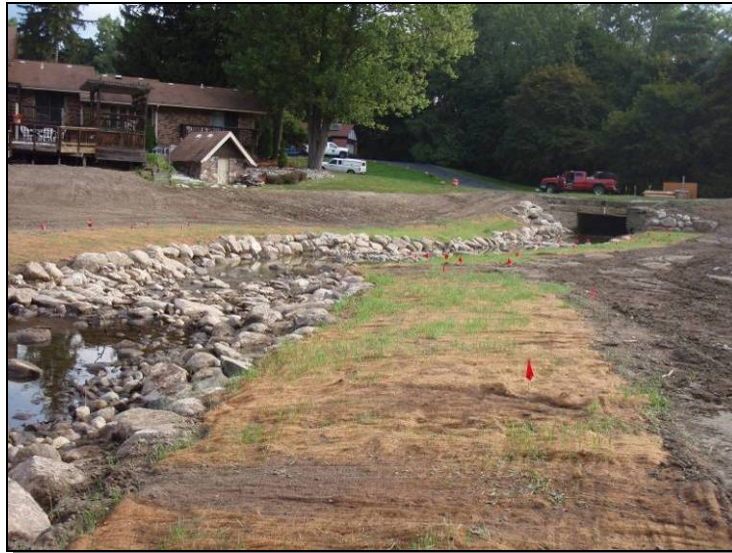
Plant locations staked
