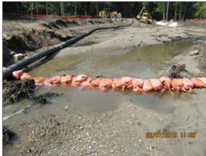
Sand bags at the downstream end of the site, just upstream from the culvert
