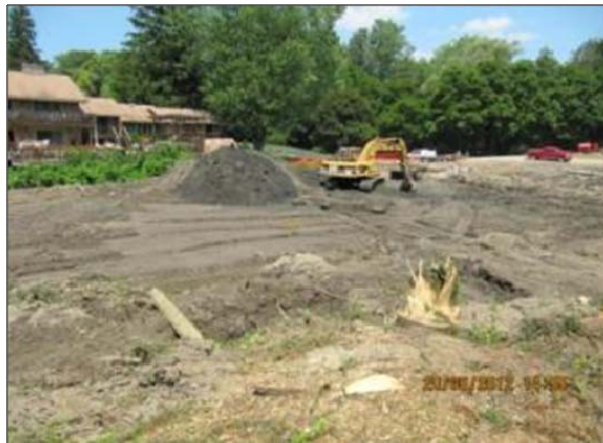
Grading at north side of pond
