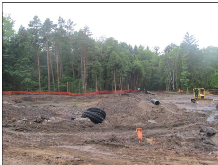
June 18, 2012: Site, view looking west, after a rain event
