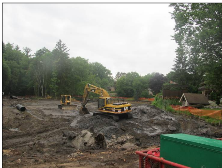
June 18, 2012: Site, view looking northwest, after a rain event
