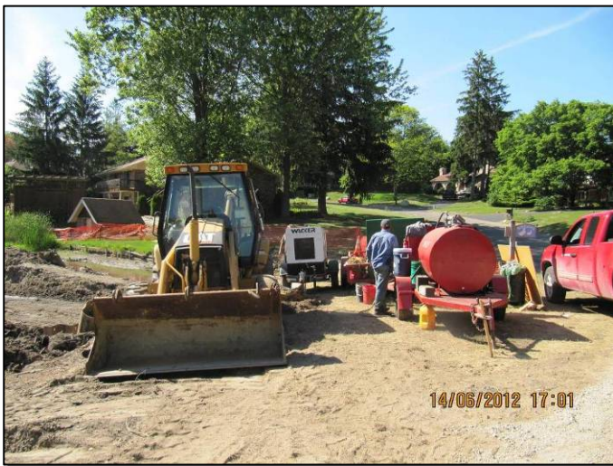
June 14, 2012: Equipment near culvert
