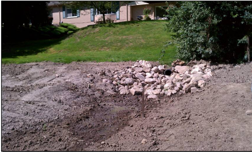
August 20, 2012: Rock apron at north sewer outfall
