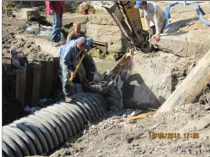
Notching at the dam for installation of bypass flume
