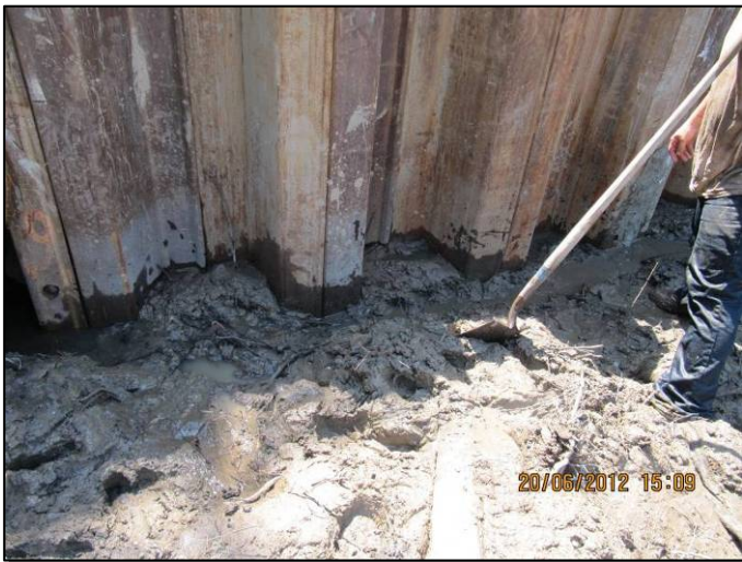
June 14, 2012: Plugging leaks in temporary dam
