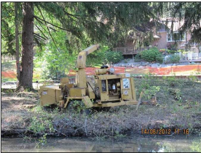
June 14, 2012: Chipper onsite
