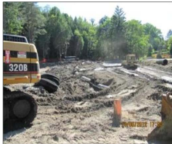
Bypass flume, view looking northwest
