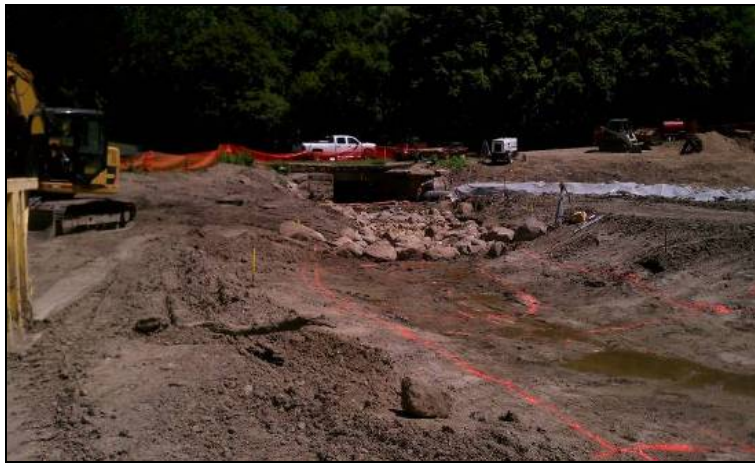
Rock placed for riffle/pool 5 and 4
