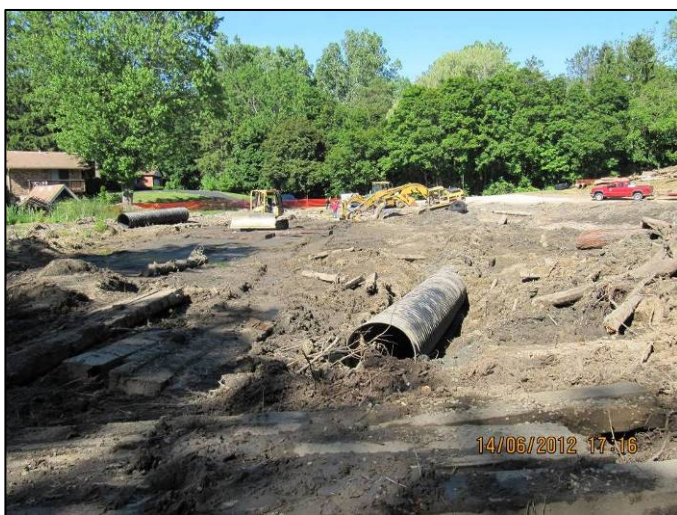
June 14, 2012: Installation of bypass flume
