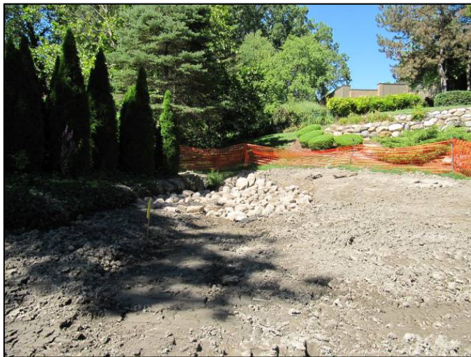
August 6, 2012: Rock Apron at west storm outfall
