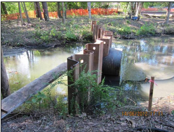
June 14, 2012: Temporary dam with tap for bypass pipe
