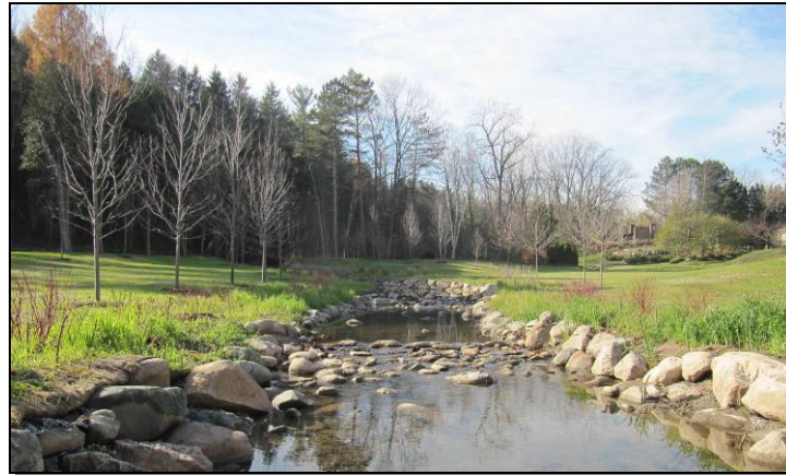
Completed Stream Channel
