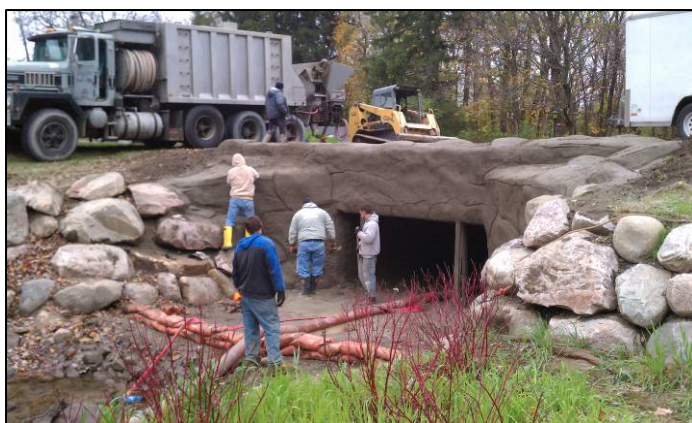
Shotcrete (Gunite) work
