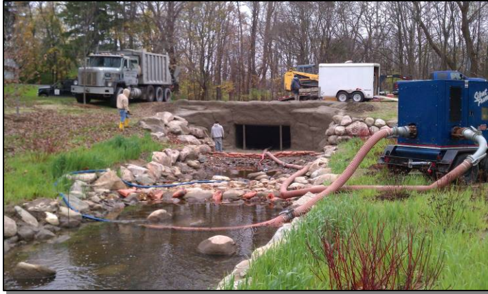
October 31, 2012: Shotcrete (Gunitite) work
