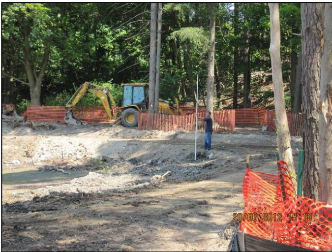
June 20, 2012: Checking grades of proposed streambank
