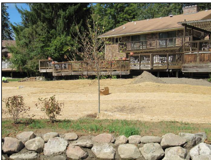
September 18, 2012: Soil pile left for homeowner
