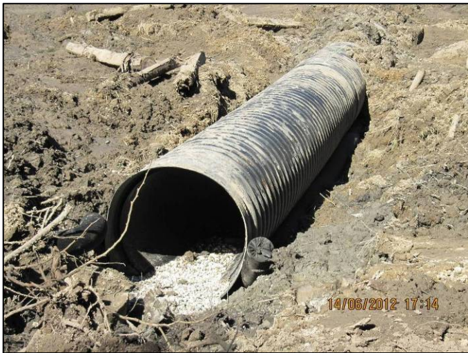
June 14, 2012: Bypass pipe with drainage along either side
