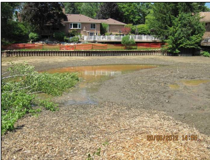
June 20, 2012: Groundwater surfacing on west side of former pond
