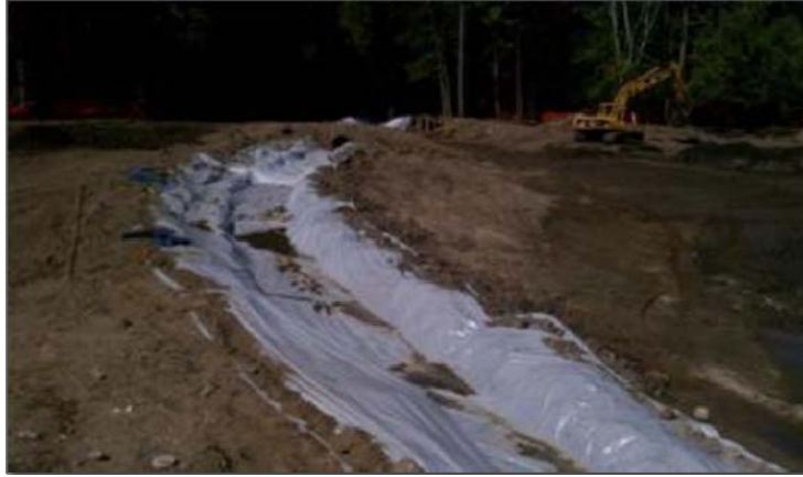
Temporary overflow channel
