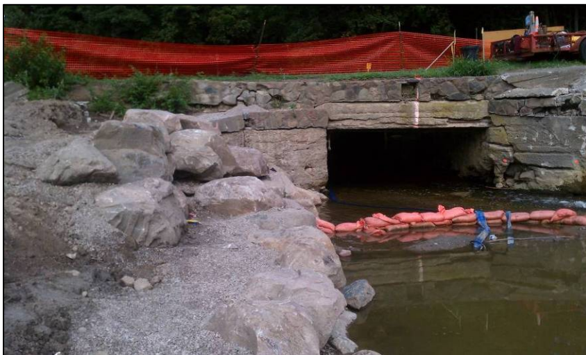
August 15, 2012: Concrete walls at culvert with boulder wall
