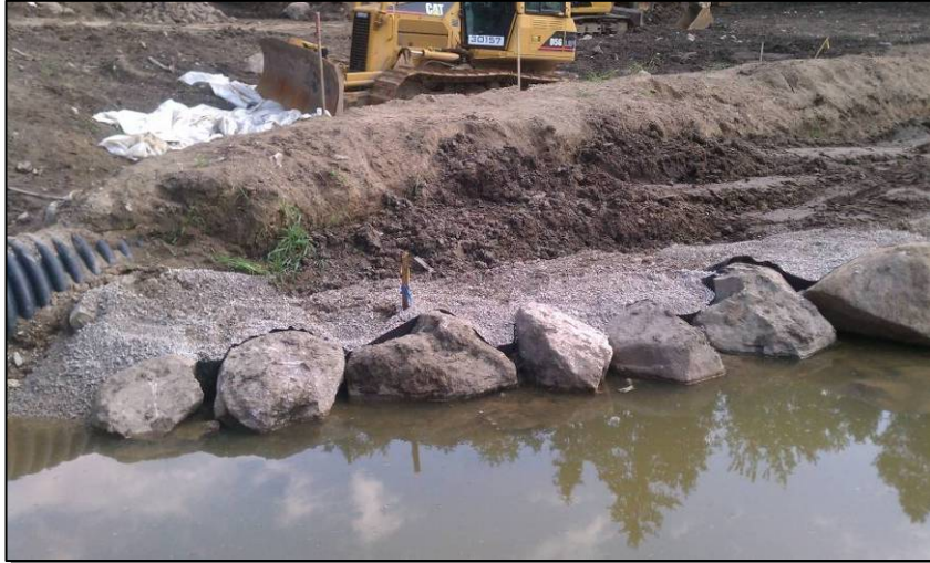
August 15, 2012: North boulder wall
