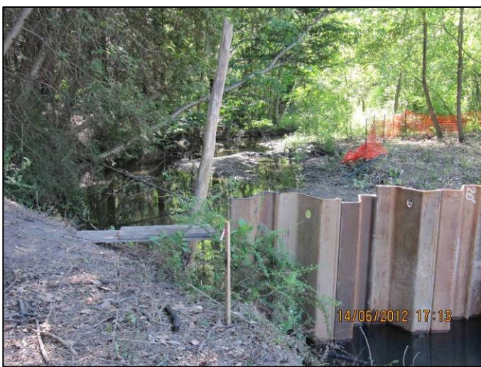
June 14, 2012: Temporary dam
