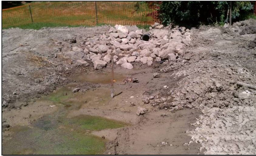
August 6, 2012: Rock apron at north storm sewer outfall
