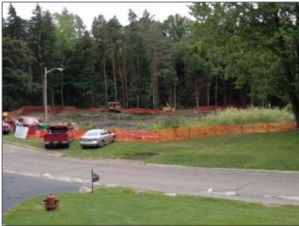
Clearing, view from across Danvers Drive, looking west
