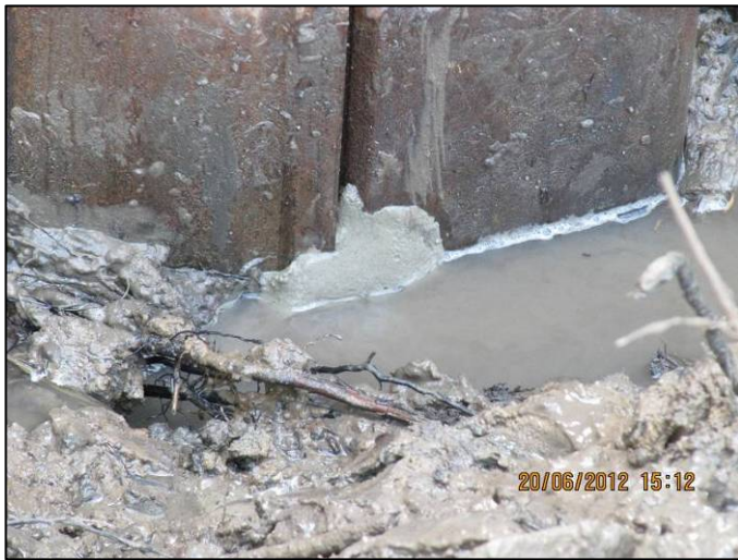
June 20, 2012: Plugging leaks in temporary dam – close up
