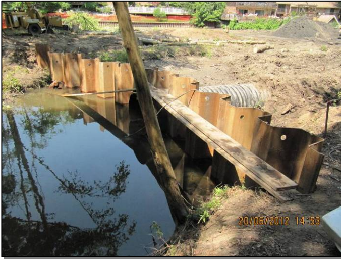
June 20, 2012: Water pumped from west side of pond to upstream of temporary dam
