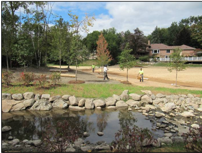
September 18, 2012: Erosion control matting
