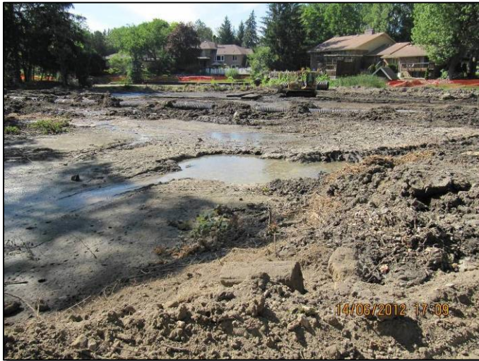
June 14, 2012: Groundwater surfacing
