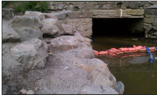
Boulders at the north bank at the culvert
