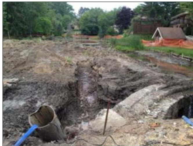
Well point installed to help with dewatering
