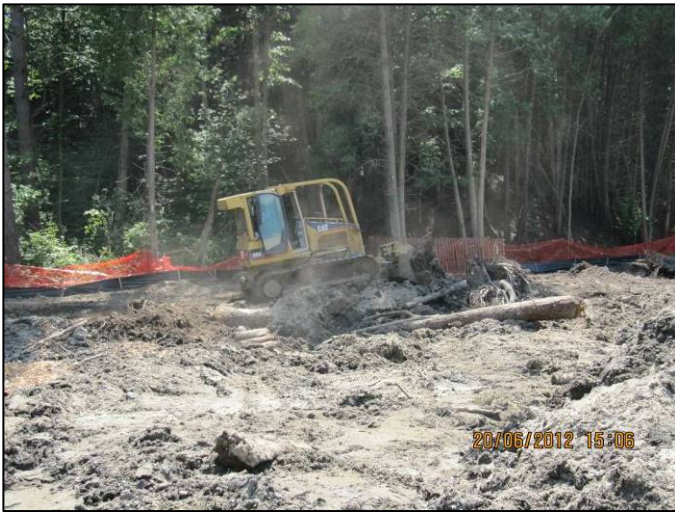
June 20, 2012: Grading the proposed streambank
