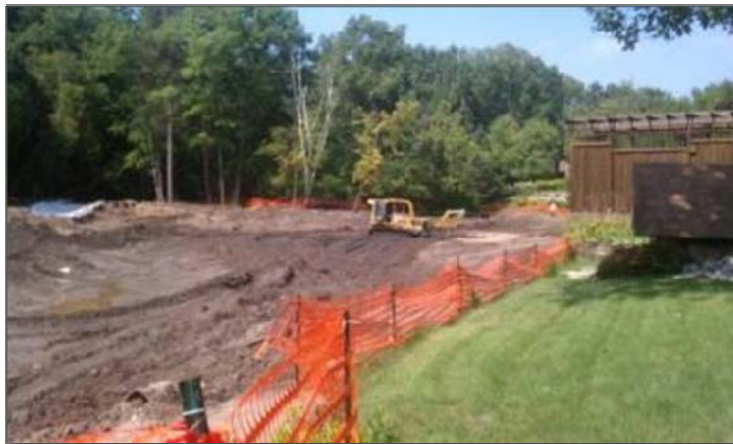
Site Grading at the north side of the site
