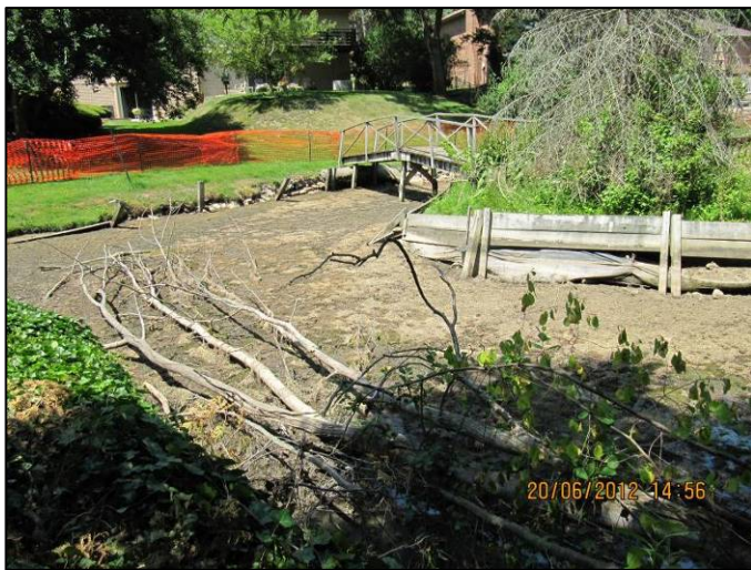
June 20, 2012: West side of pond – completely dredged
