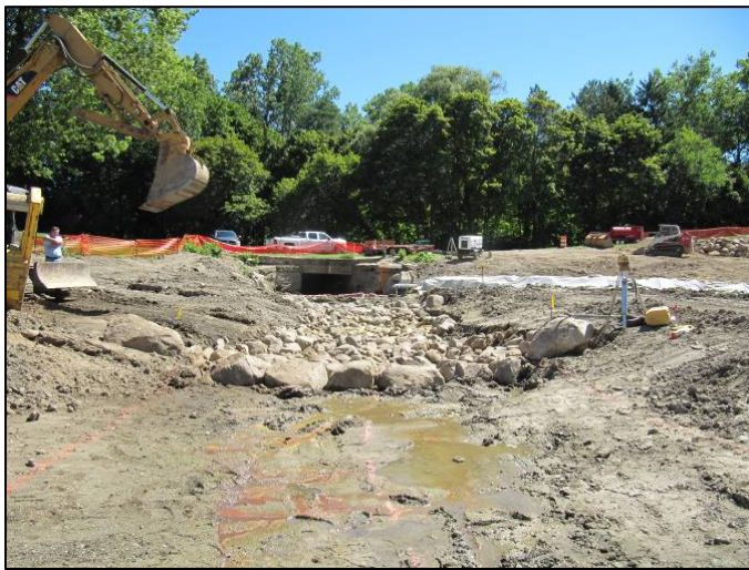
August 6, 2012: Crew working on Riffle crest 4
