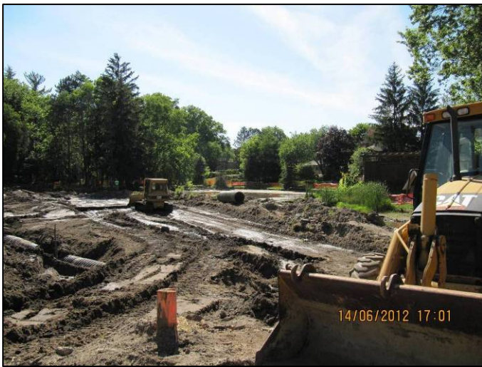
June 14, 2012: Site work, view looking north
