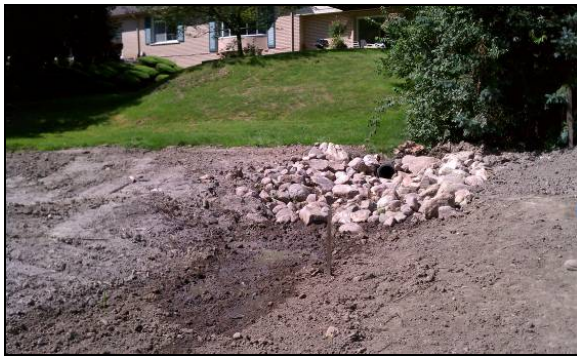
Rock at the north storm sewer outfall
