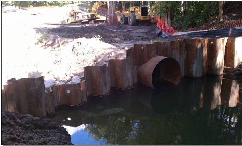
August 20, 2012: Coffer dam
