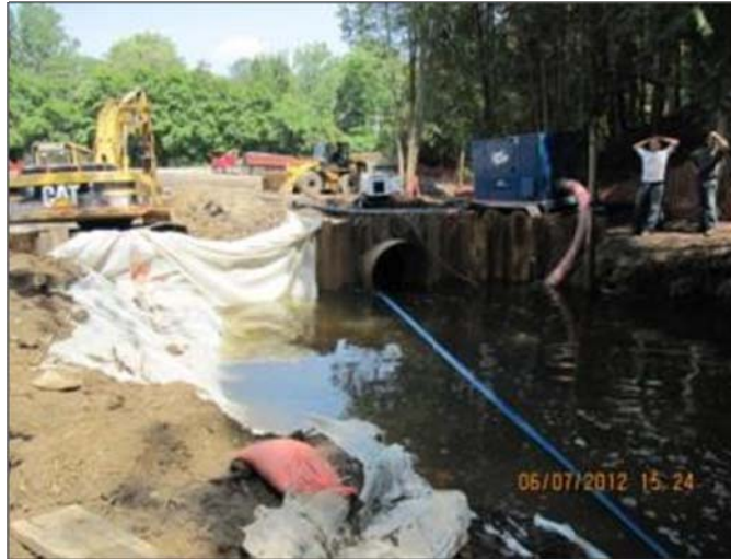
Upstream side of cofferdam, note pumping
