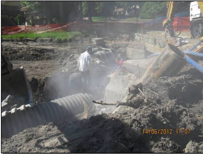
June 14, 2012: Cutting concrete
