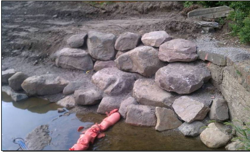
August 15, 2012: North boulder wall
