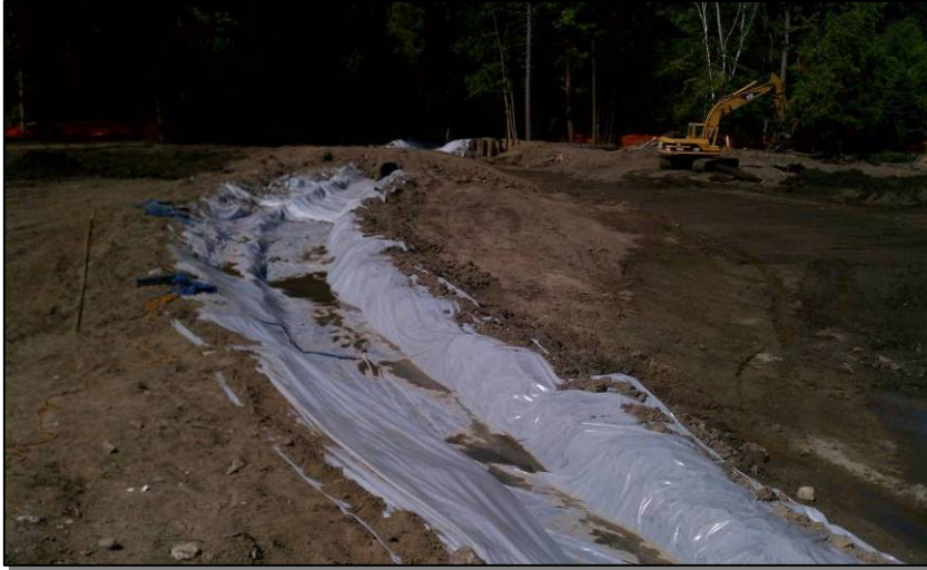
July 11, 2012: Temporary emergency spillway channel
