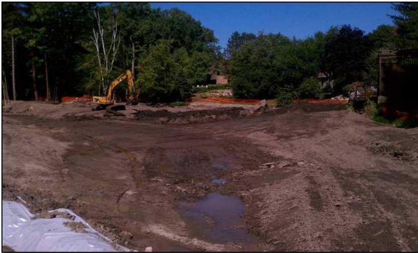
July 11, 2012: Excavating/grading at the north end of site
