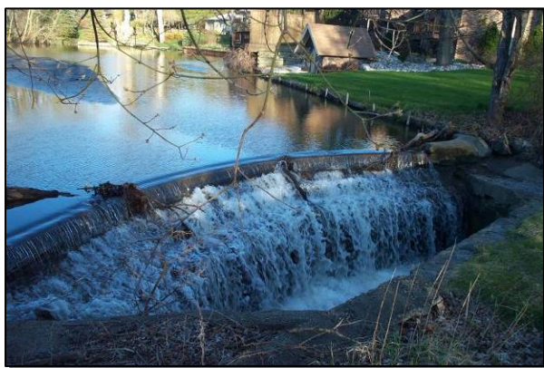
Danvers Pond Dam prior to project implementation
