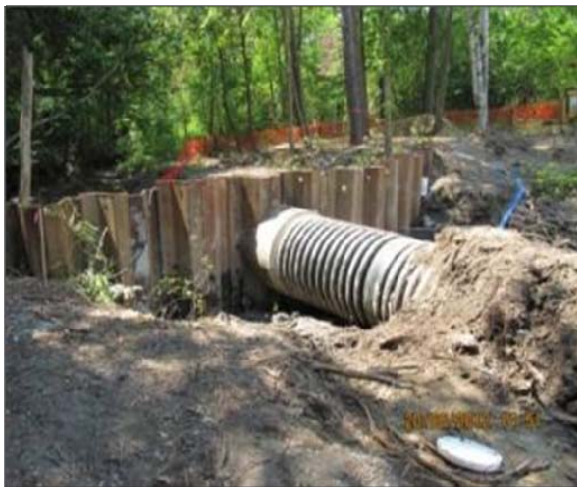
Cofferdam and connected bypass flume
