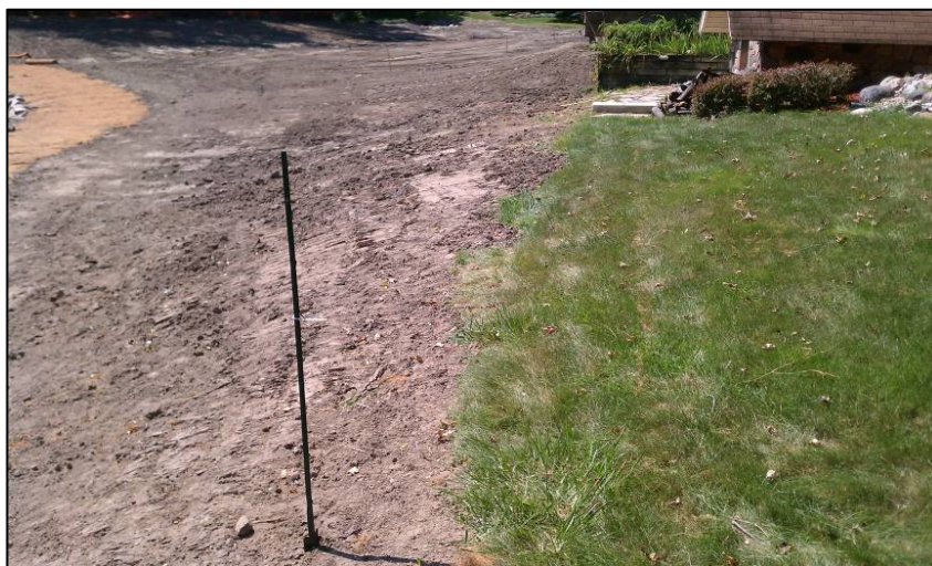
August 23, 2012: Drainage pipe outlet from east property
