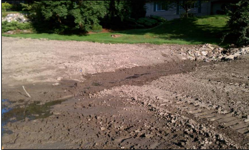
August 22, 2012: Swale near north storm water outfall
