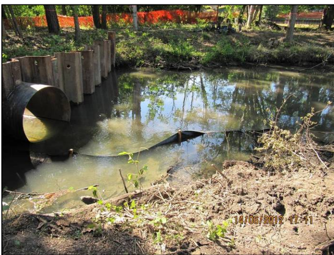
June 14, 2012: Temporary dam with erosion fence
