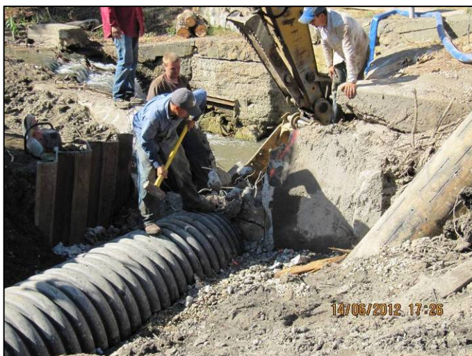
June 14, 2012: Demolishing dam to make room for bypass pipe
