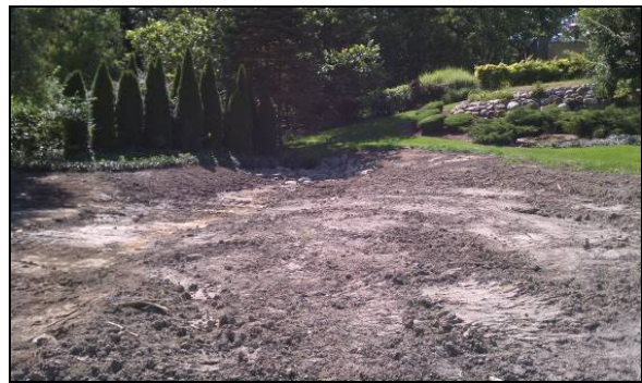
Rock at the northwest storm sewer outfall
