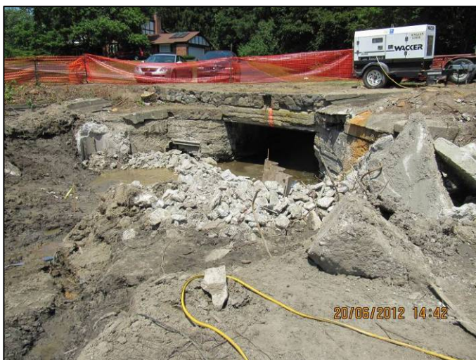
June 20, 2012: Demolished dam
