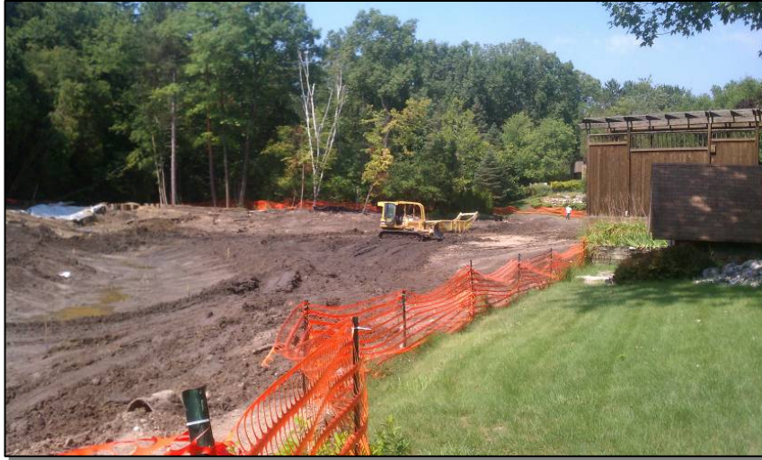
July 30, 2012: North end of site, placing rock aprons
