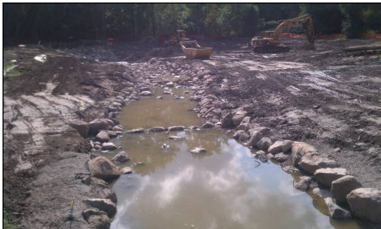
Stream channel, view looking upstream (west)
