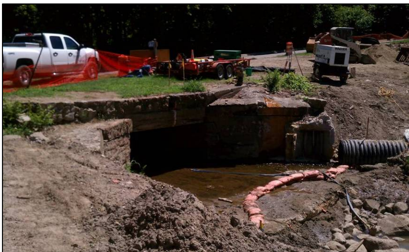
August 6, 2012: Concrete walls at end of culvert
