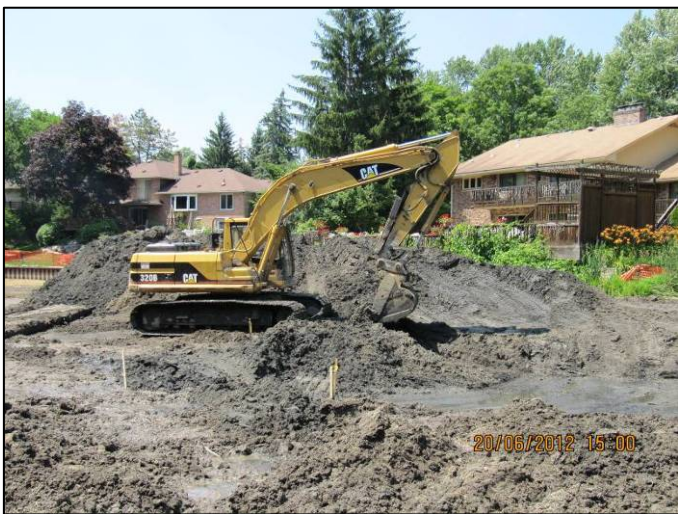
June 14, 2012: Excavation of proposed channel
