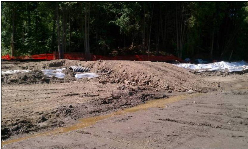
July 11, 2012: Access Road over temporary emergency overflow
