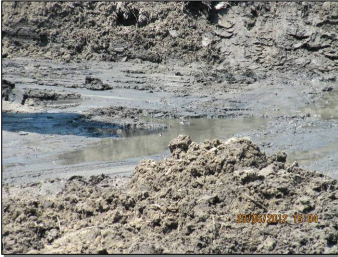
June 20, 2012: Groundwater surfacing as channel is being excavated
