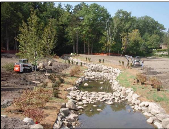
September 6, 2012: Installation of trees shrubs
