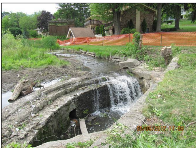
June 5, 2012: Looking southwest over dam
