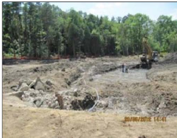
Grading for proposed channel
