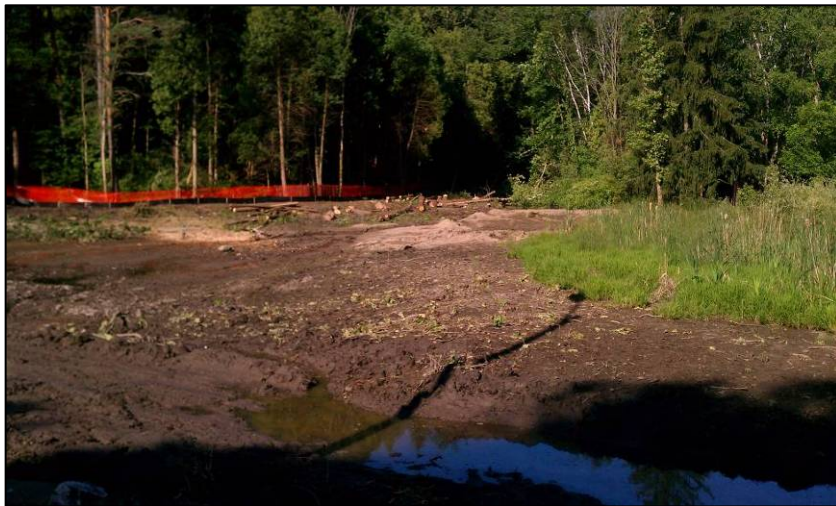
June 7, 2012: View looking west, from road embankment
