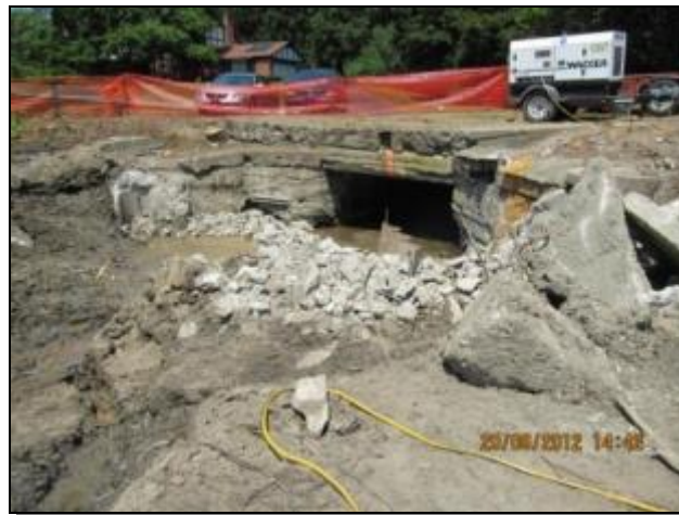
Dam spillway removed
