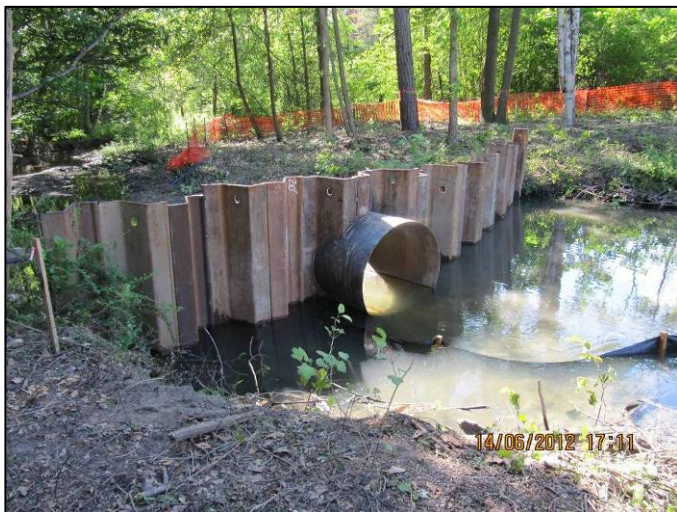
June 14, 2012: Sheet pile cofferdam with pipe stub.
