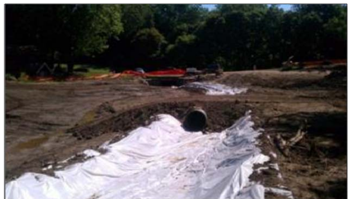
Temporary overflow channel
