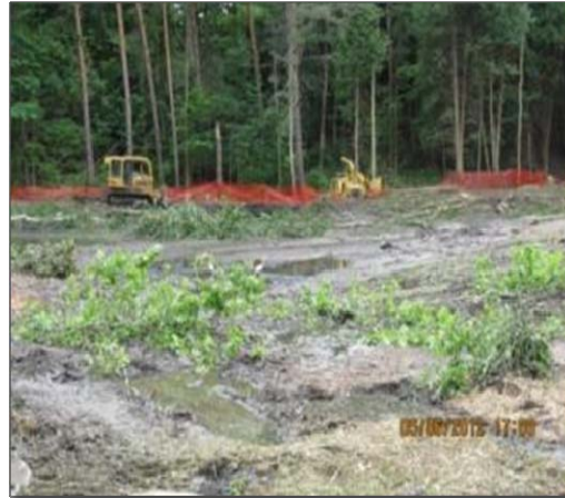
Clearing, view looking west
