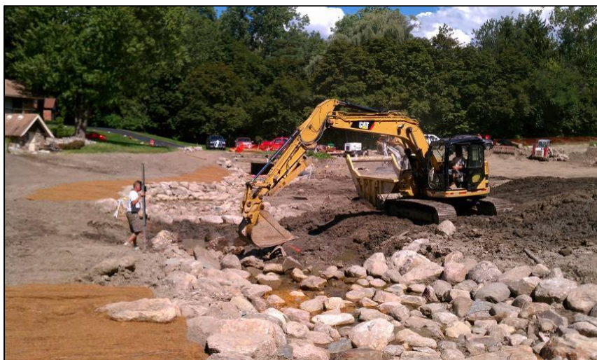
August 20, 2012: Riffle 2 construction
