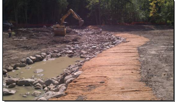
Work at riffle/pool 2, view looking east, note stream bank constructed north bank
