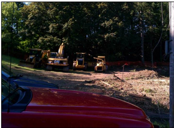
June 7, 2012: South side of site, equipment staged
