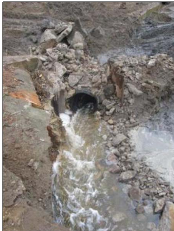
Water flowing through the bypass flume
