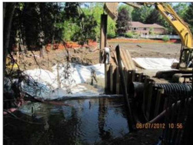
Installation of additional sheet piles at north end of cofferdam
