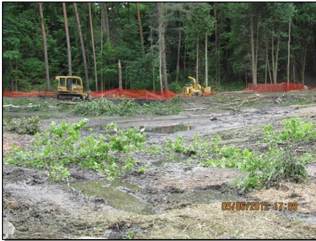
June 5, 2012: Clearing, view looking south
